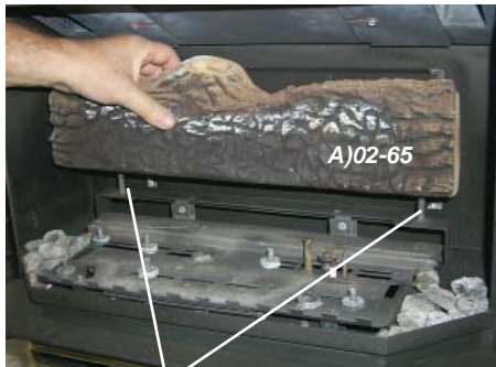
Pins on Rear Log Support
